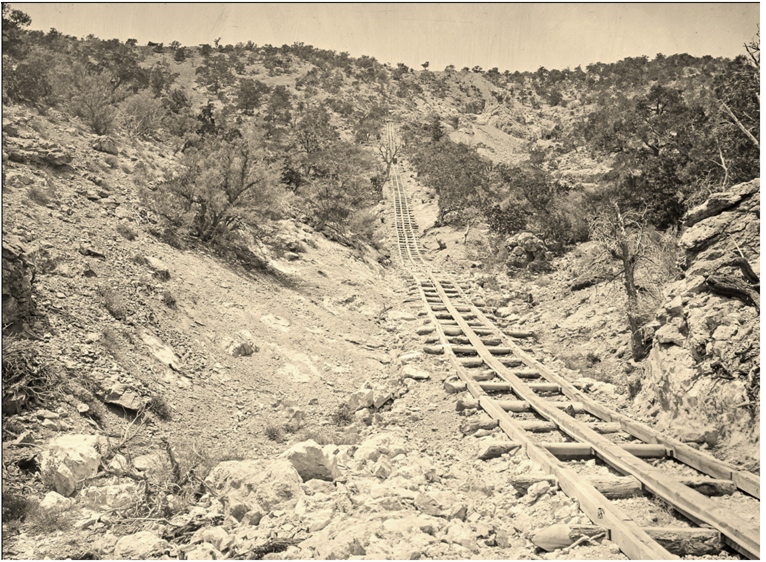
14 A wooden balanced incline used for gold mining, at the Illinois Mine in the Pahrangat Mining District, Nevada in 1871. An ore car would travel on the parallel tracks connected to a pulley wheel at the top of tracks. (Timothy O'Sullivan/National Archives and Records Administration) #
